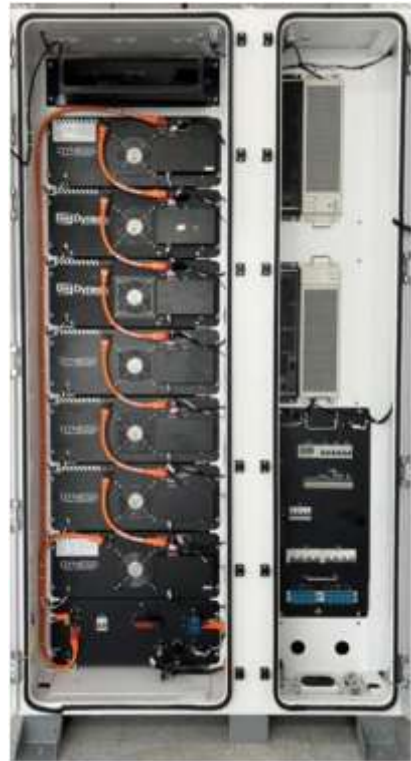
⑥ Series the battery packs
